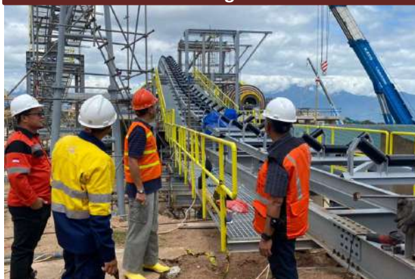
Conveyor to feed ores from crusher to milling unit
