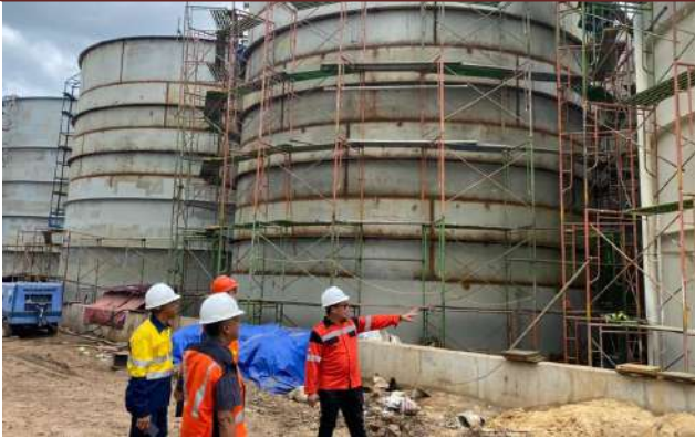
Carbon in Leach Tanks have been installed
