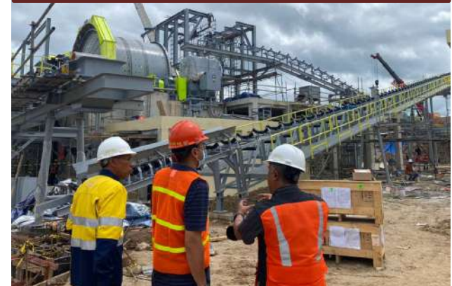
Conveyor to feed ores from crusher to milling unit
