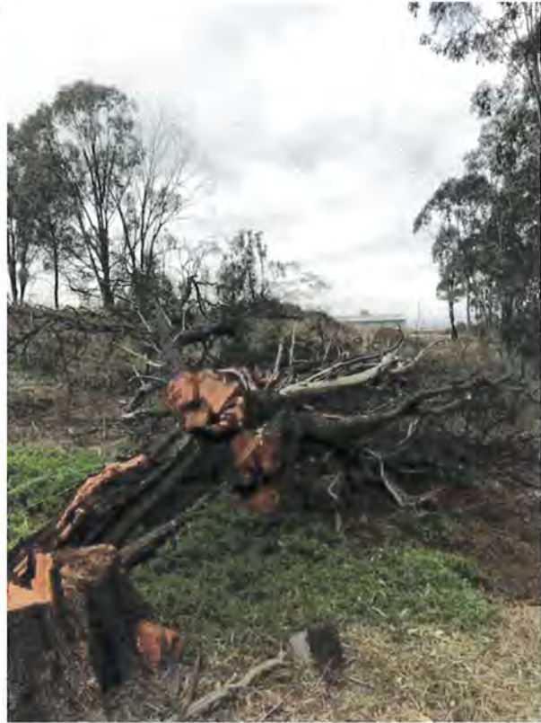
Photo 3.6 Stage 2 – clearing – post felling
