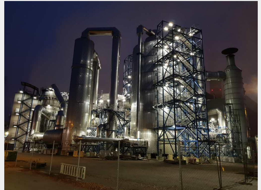
Acid plant Harjavalta
