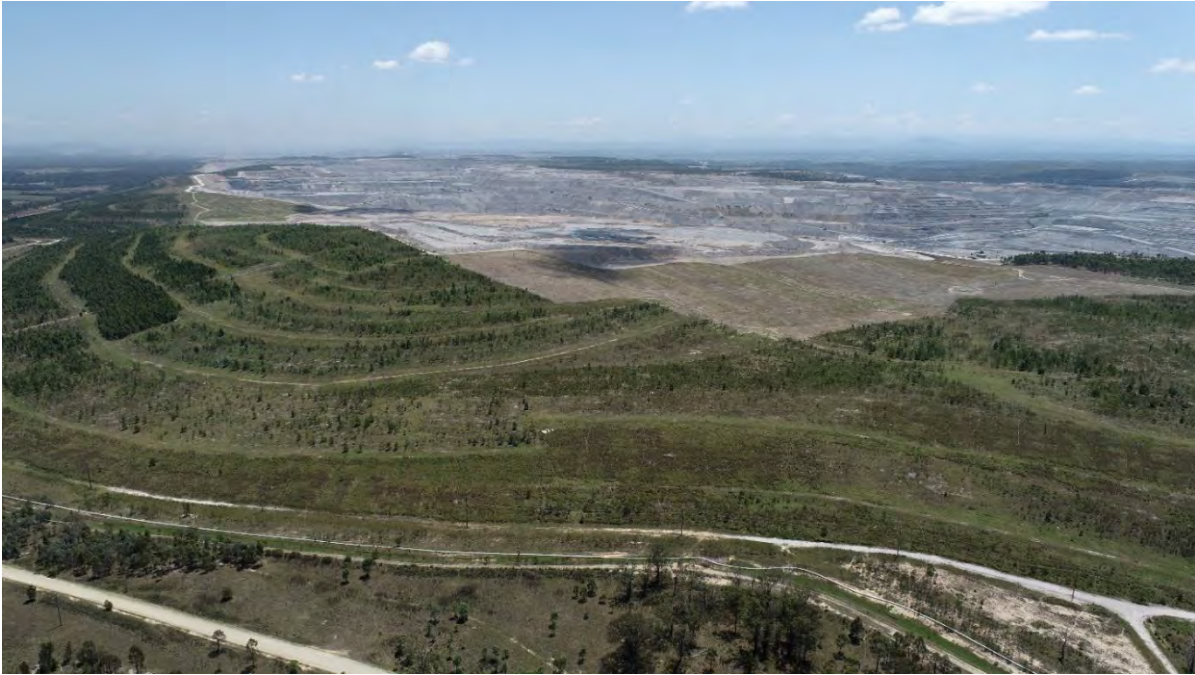
Photo 3 Rehabilitation completed in 2022 surrounded by previously rehabilitated areas on the Noise and Visual Bund
