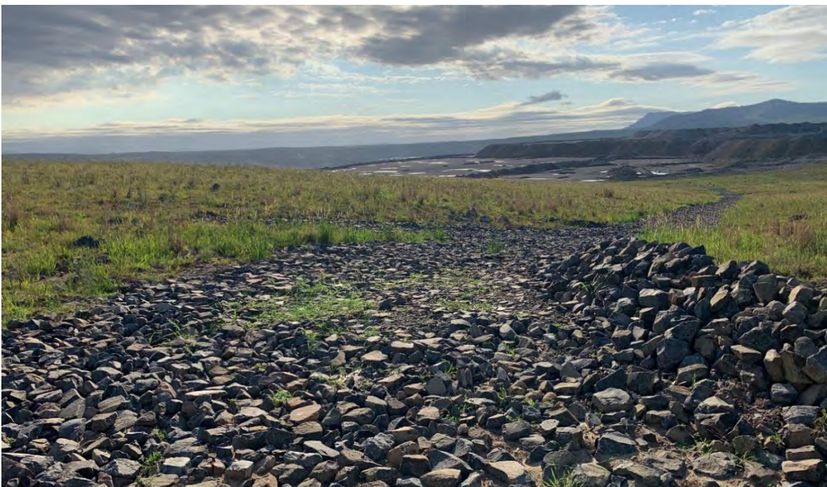
Photo 4 Constructed geomorphic landform drainage on the Noise and Visual Bund in 2022
