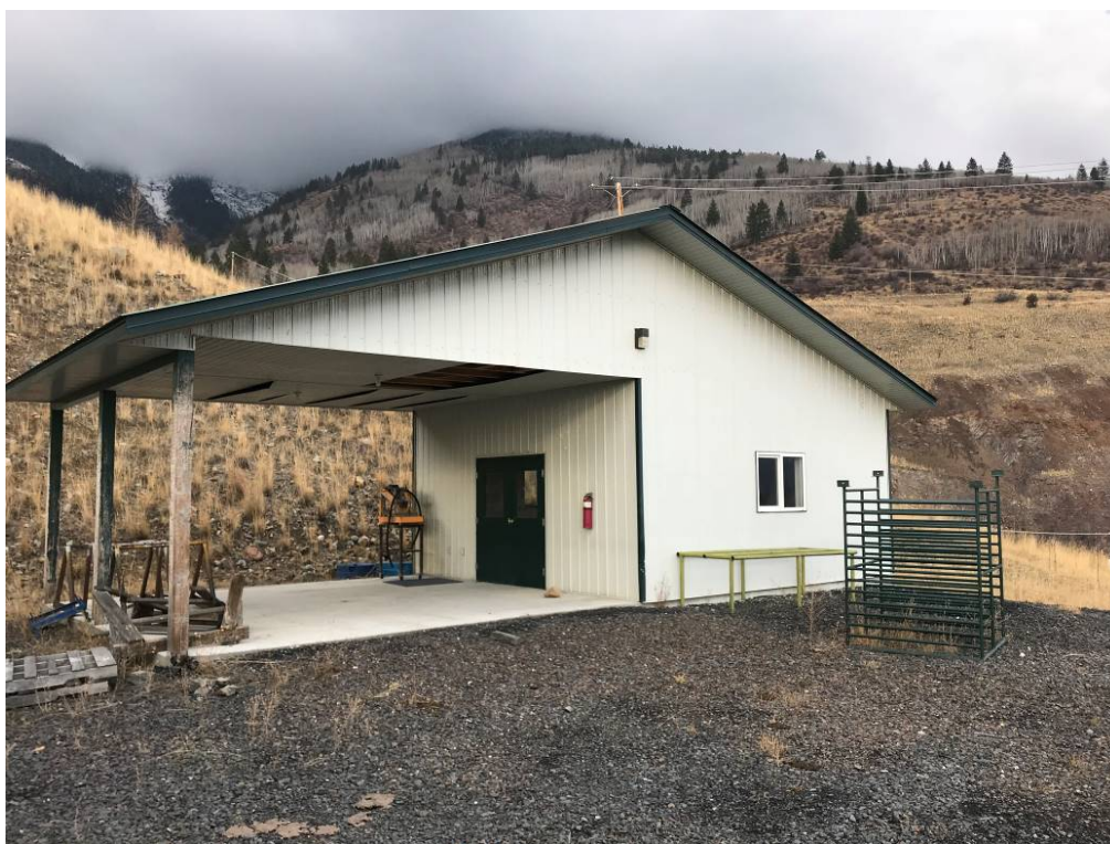
Figure 12-2 Mine Site Core Cutting Shed (Source: MMTS 2021)
