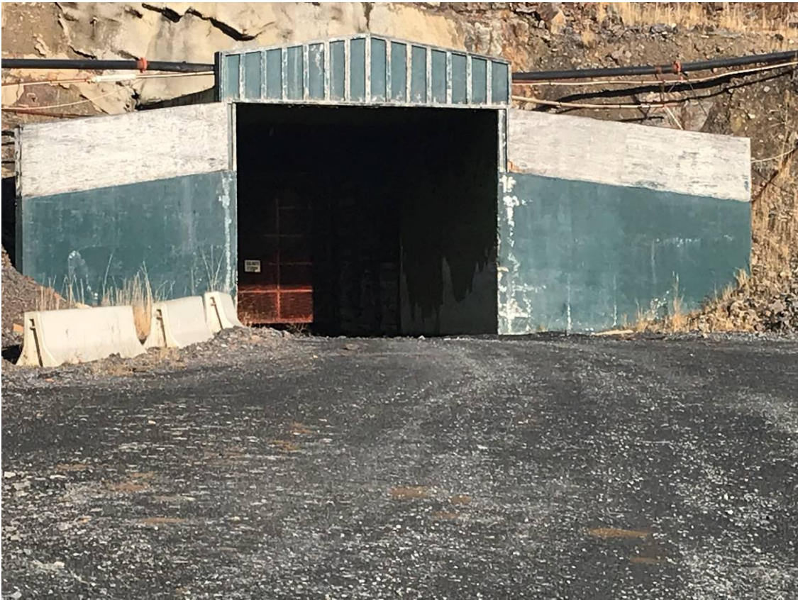
Figure 11-35 Locked Entrance to the Underground Workings (Source: MMTS 2019)
