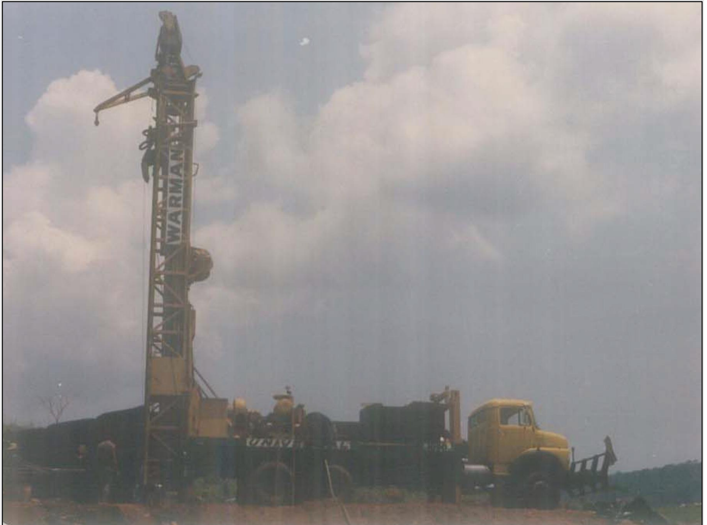
Figure 6-10: Warman Rig in Operation on The Cabaçal Deposit, São Paulo Farm.
