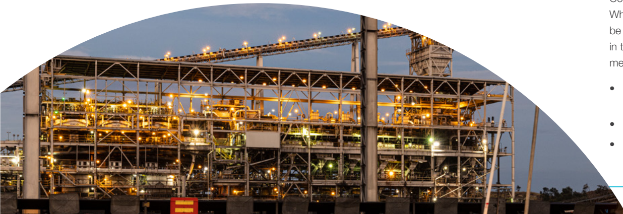
CHPP at Curragh mine
