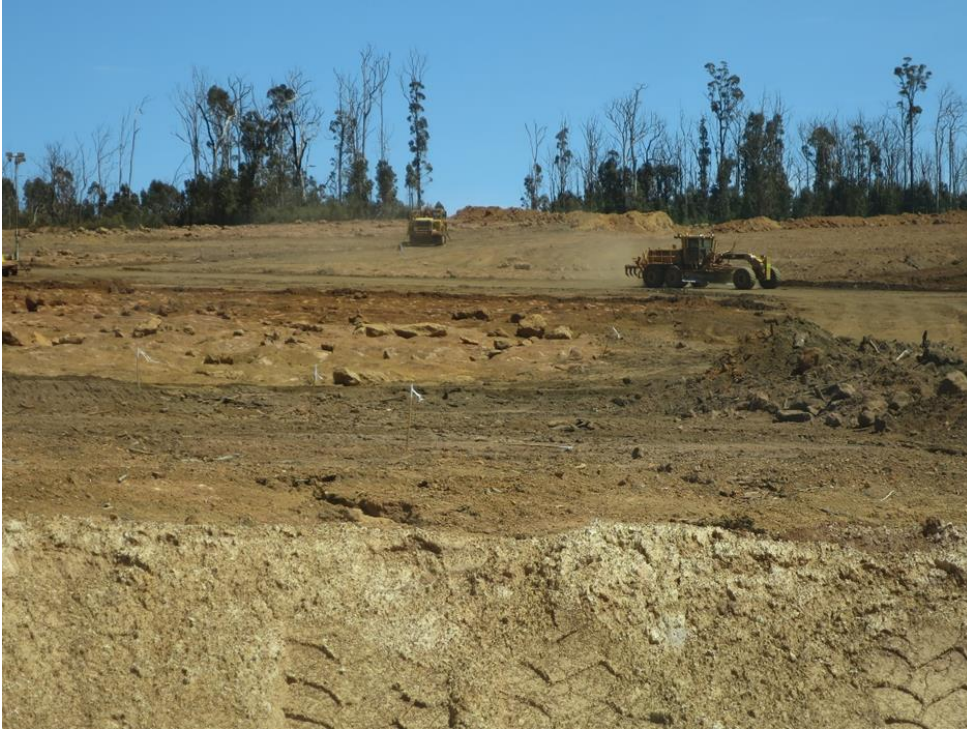
Figure 13-2: Topsoil Removal (Background), Blasting of Hardcap and Marking of Ore (foreground) (SLR, 2021)
