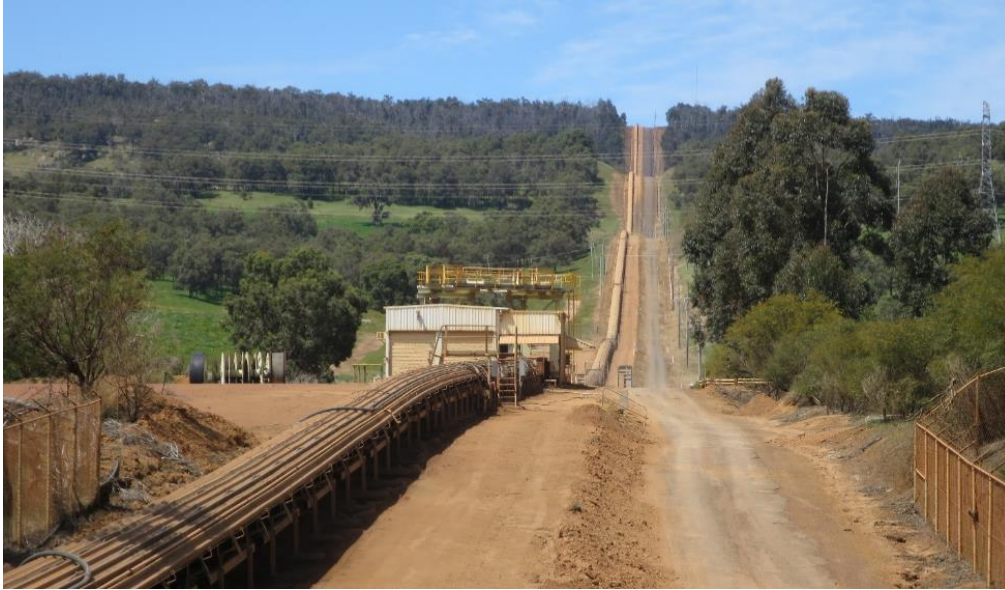
Figure 13-6: Covered Conveyor (SLR, 2021)
