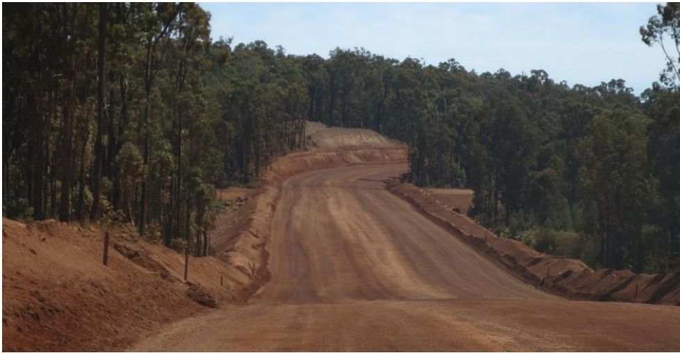
Figure 13-5: Haul Roads with Berms (SLR, 2021)
