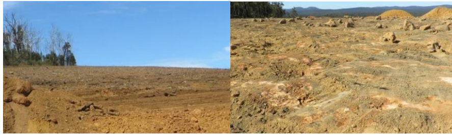
Left: Vegetation cleared prior to mining. Right: Top soil and oxalate removed leaving Hardcap
