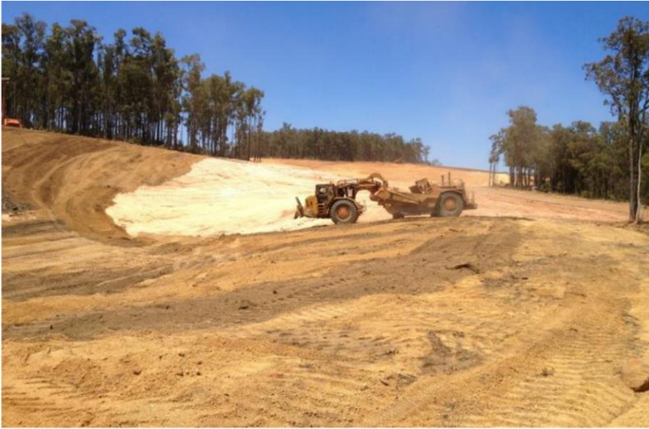
Figure 13-8: Soil Being Returned for Backfilling and Landscaping the Pit (Alcoa, 2018)
