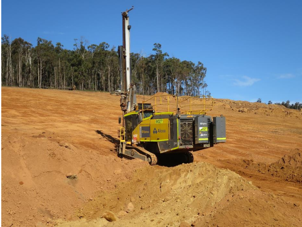
Figure 13-12: Blasthole Drill Working on Hardcap (SLR, 2021)
