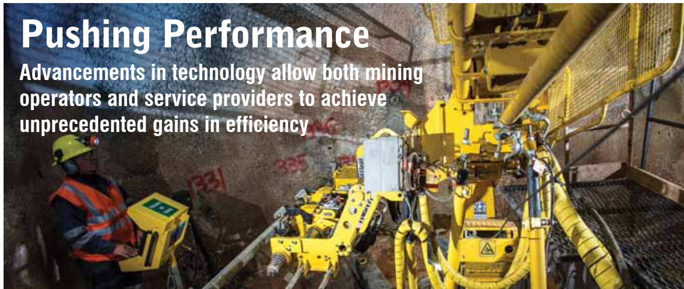
Drilling contractors have been incorporating new technologies for productivity and safety. Photo courtesy of Geotec.
