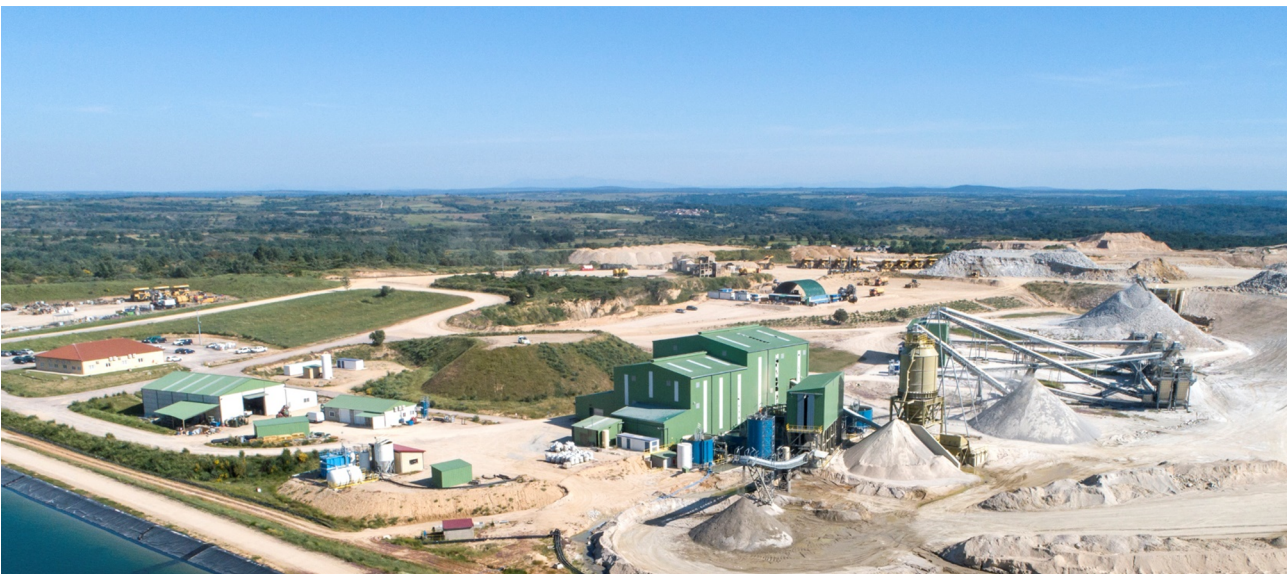
Fig.3 - Barruecopardo Site: Looking from North to South; in front the main processing plant with the crushing & screening circuits to the right
