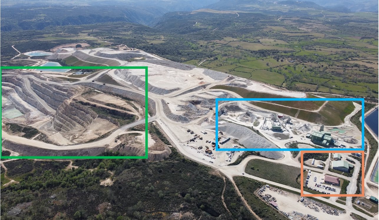
Fig.2 - Barruecopardo Site: In Green shown the mining operation, in Blue shown the crushing & screening circuits and main processing plant; in Orange shown the laboratory and administration building
