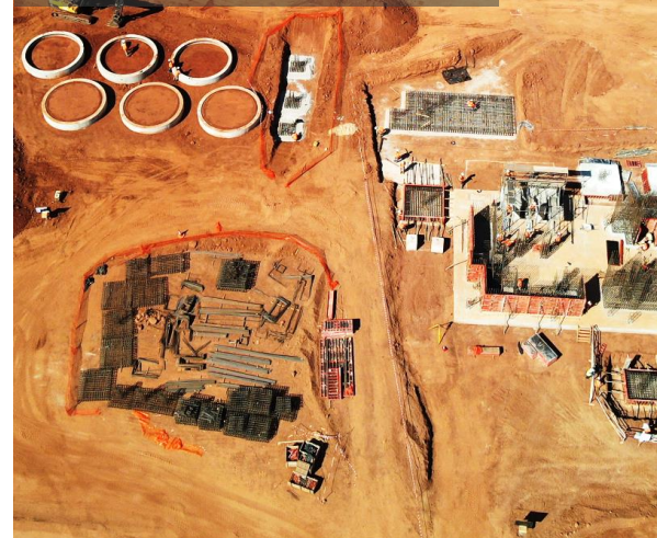
CIL Tanks and SAG + Ball mill construction
