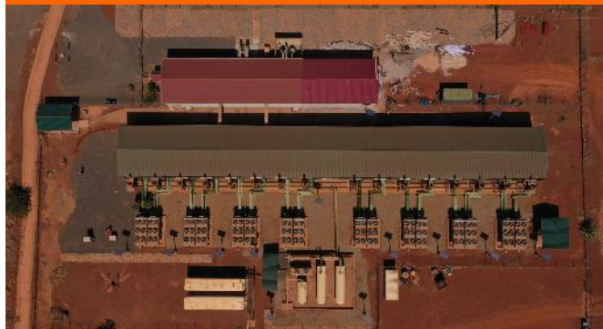
26MW Back-up Power Station
