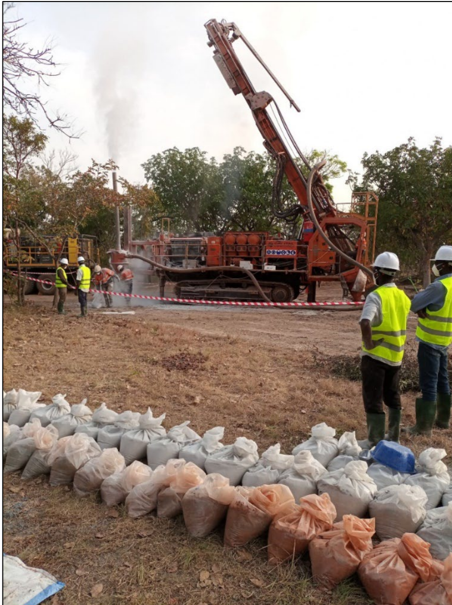
Drilling at Goulamina
