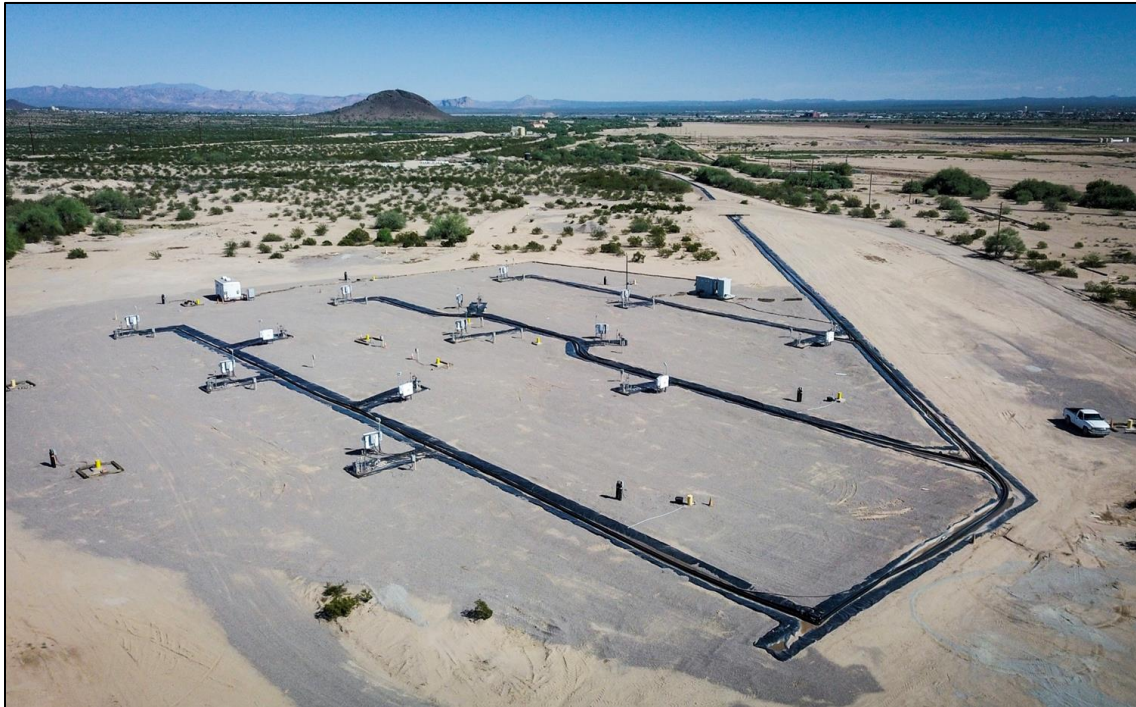
Figure 13-8: Aerial View of PTF Well Field
