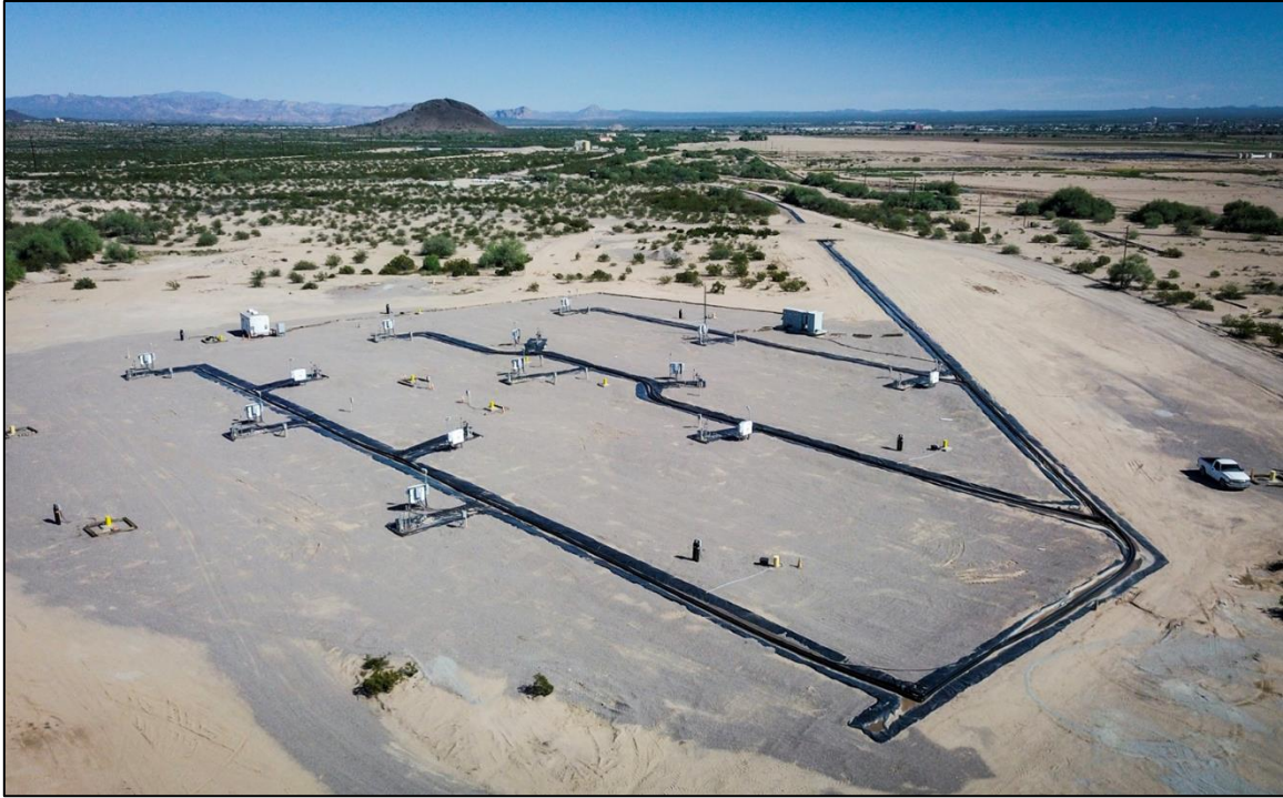
Figure 16-1: Aerial Photo of Florence Copper PTF Well Field
