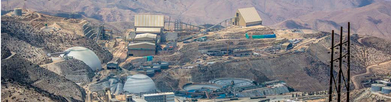
Following a US$1.3 billion investment, Toquepala has doubled its processing capacity from 60,000 mt/d to 120,000 mt/d. Photo courtesy of Southern Copper.
