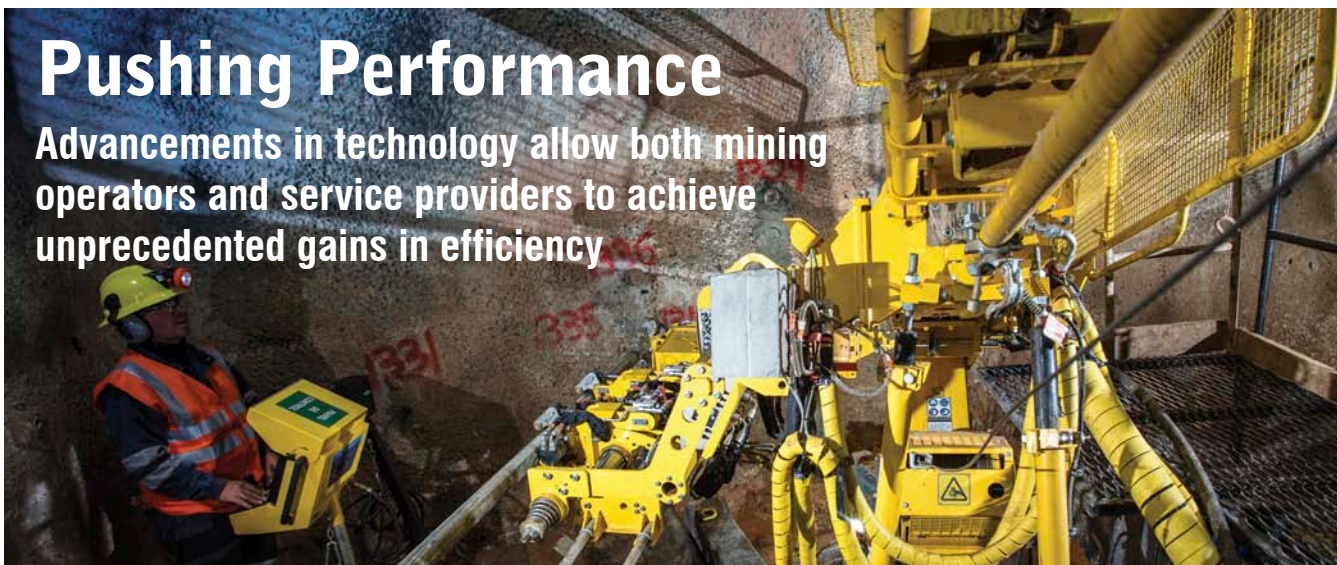
Drilling contractors have been incorporating new technologies for productivity and safety. Photo courtesy of Geotec.
