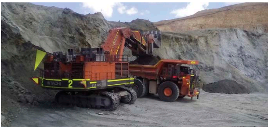
Hitachi equipment doing early works at Mina Justa. Photo courtesy of Zamine.
