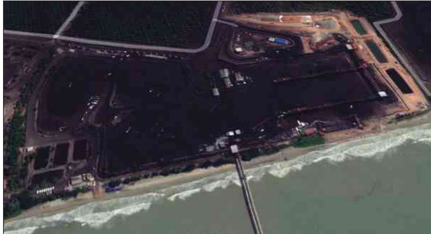
Figure 8:4 Coal Loading Facilities at Port
