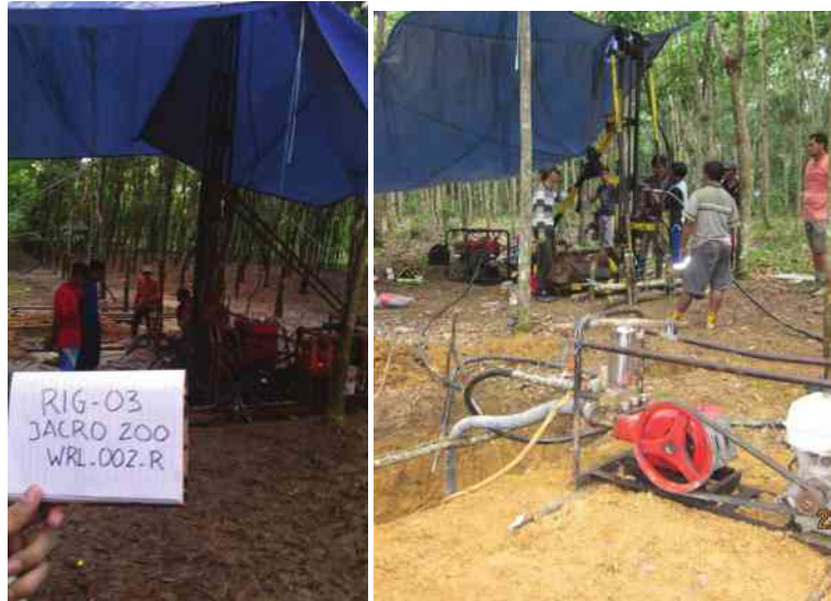
Figure 3:3 WRL Drilling Operations
