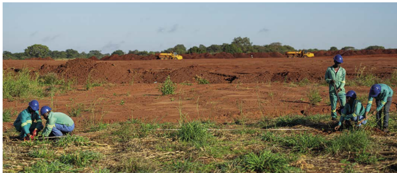
IMAGE Back-filling and post environmental rehabilitation, Montepuez Ruby Mining, Mozambique
