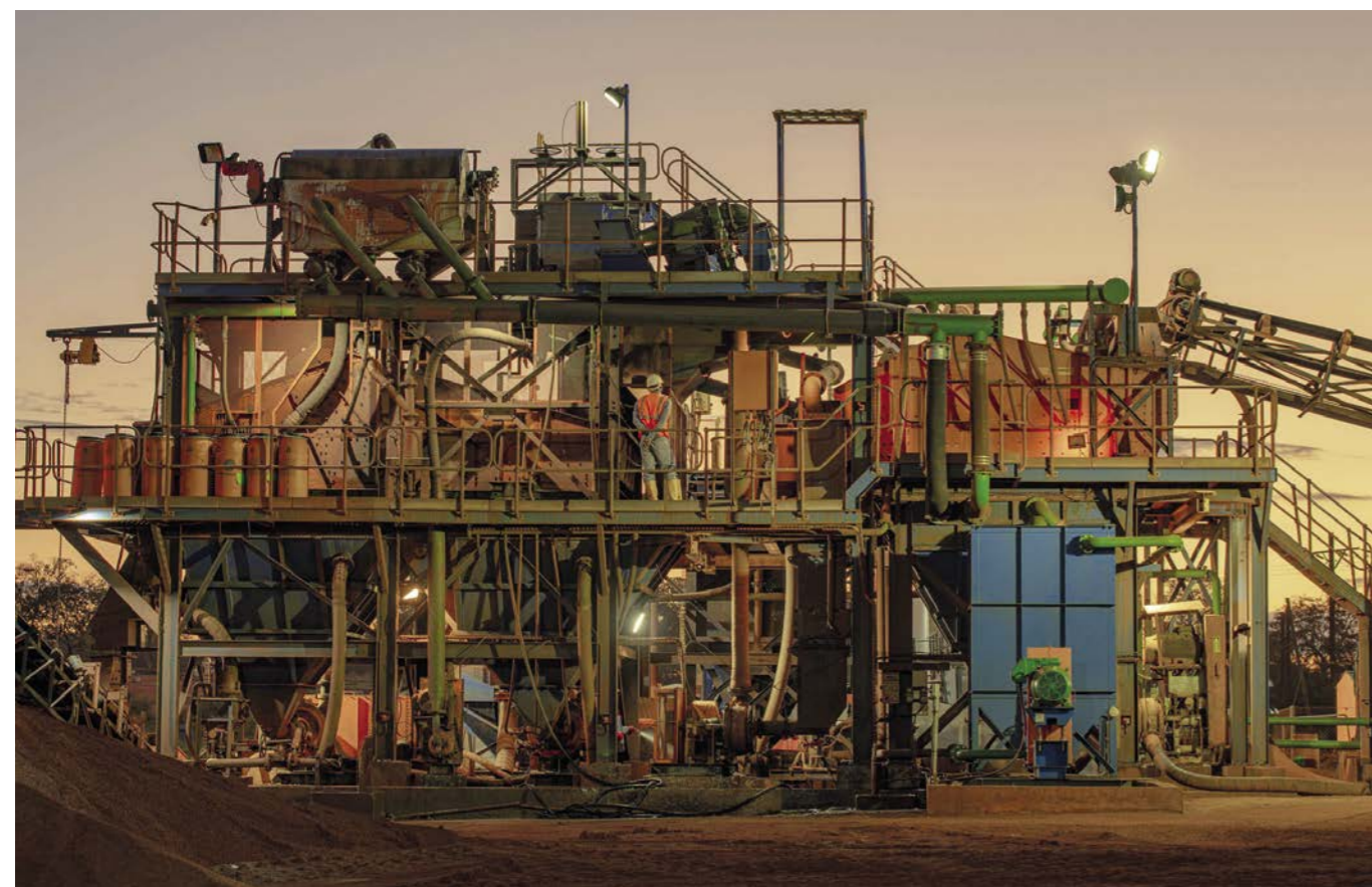
IMAGE Ruby wash plant, Montepuez Ruby Mining, Mozambique
