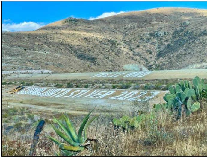
(Mastrantos IIIb - the current active tailings area at El Cubo)
