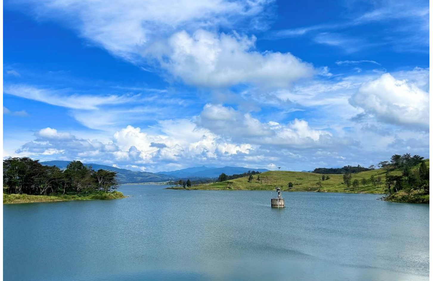
Aerial of Yonki Dam reservoir, which is the primary source of hydroelectric power for the Ramu 1 power station in PNG, from which we source our grid electricity at Kainantu.
