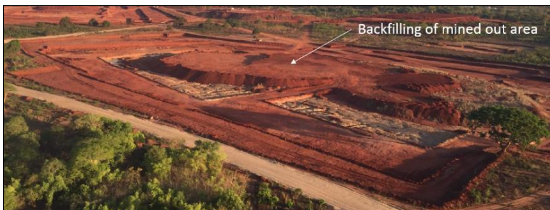
Figure 3-30: MRM: Backfilling of mined out area
