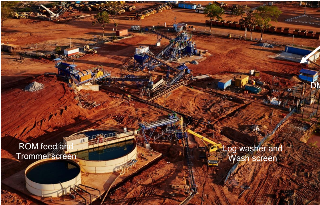
Figure 3-33: MRM: Plant layout
