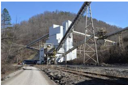
Figure 1. Kanawha Eagle preparation plant.
