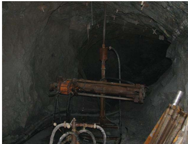
Photo 5.1: LPS-3U Pneumatic Drillrig in Operation
