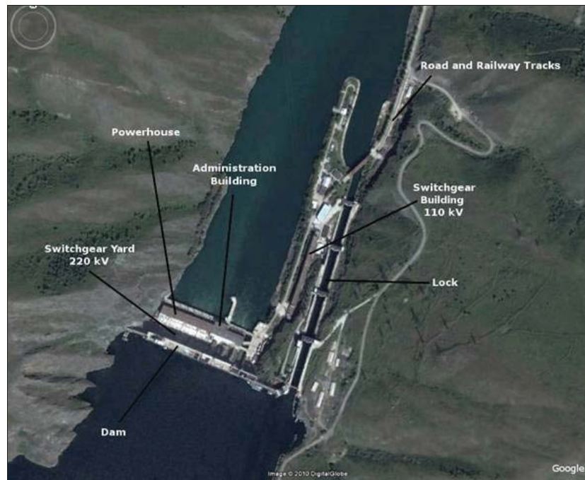
Figure 20.1: Aerial view of the Bukhtarma Hydro Plant
