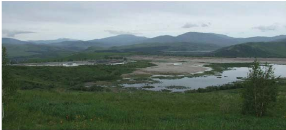
Photo 12.1: General View of the Chashinskoye Tailings Dam (looking northeast)
