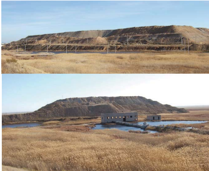
Photo 3.2: Old Heap Leach Dumps and Associated Infrastructure
