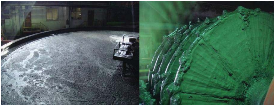
Photo 5.6: Thickening and Filtration
