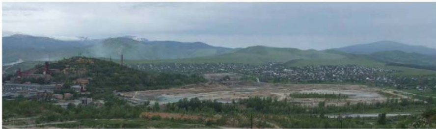
Photo 11.1: North-West view over the Staroye Tailings Dam (Ridder Concentrator to the left of the image)
