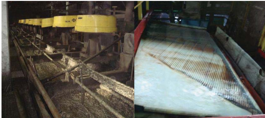
Photo 5.5: RIF Flotation Cells and Shaking Table
