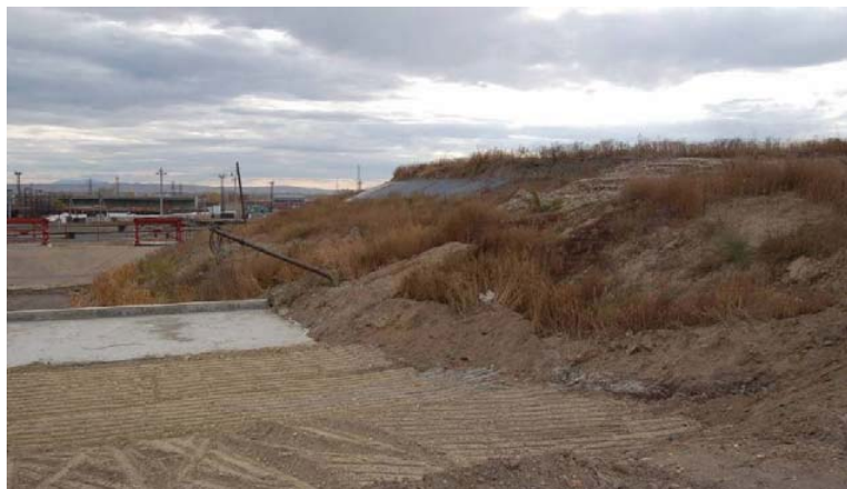
Photo 16.4: Historic Capped Calcium Arsenate Stockpile Showing Instability on Cap
