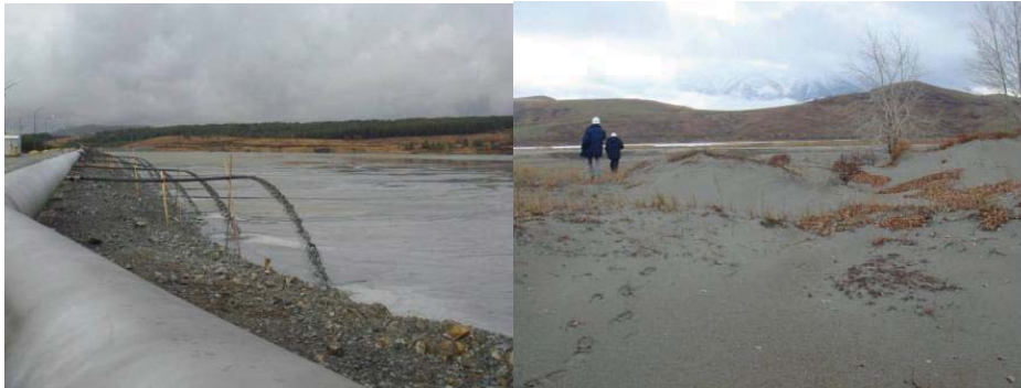
Photo 5.7: Talovskoye and Chashinskoye Tailings Dams
