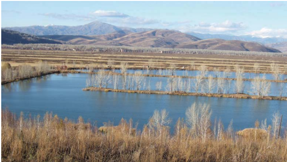
Photo 4.4: Biological (Oxidation) Water Clarification Lagoon at the TMF
