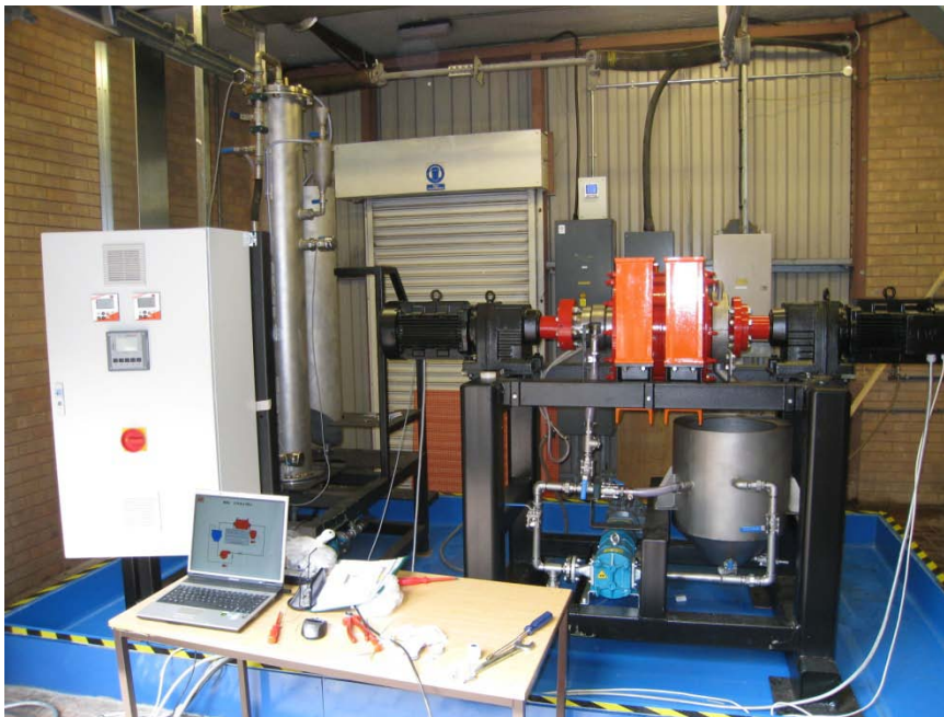
Figure 5.0 Ultra Fine Grinding Milling Pilot Plant
