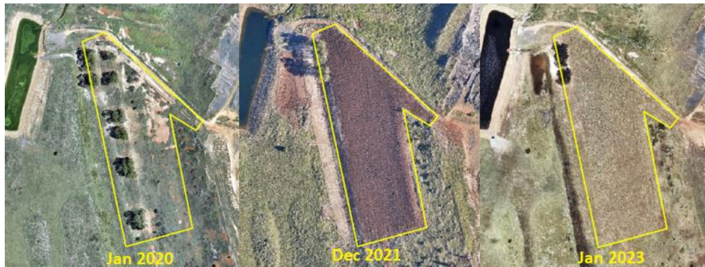
Figure 25 E22 waste rock batter rehabilitation repairs from 2020 to 2023
