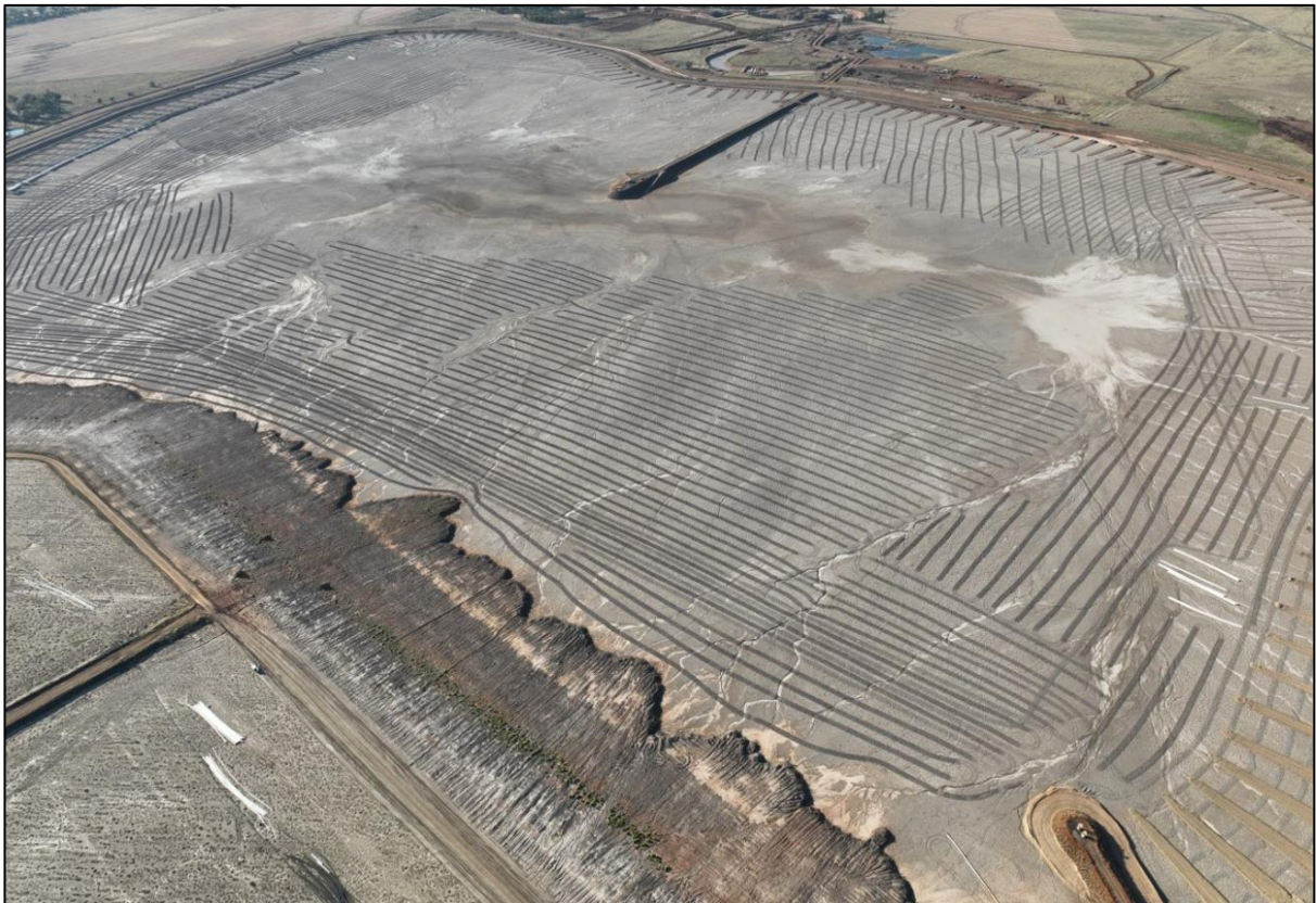
Figure 9 Ripping undertaken on Rosedale TSF for dust control
