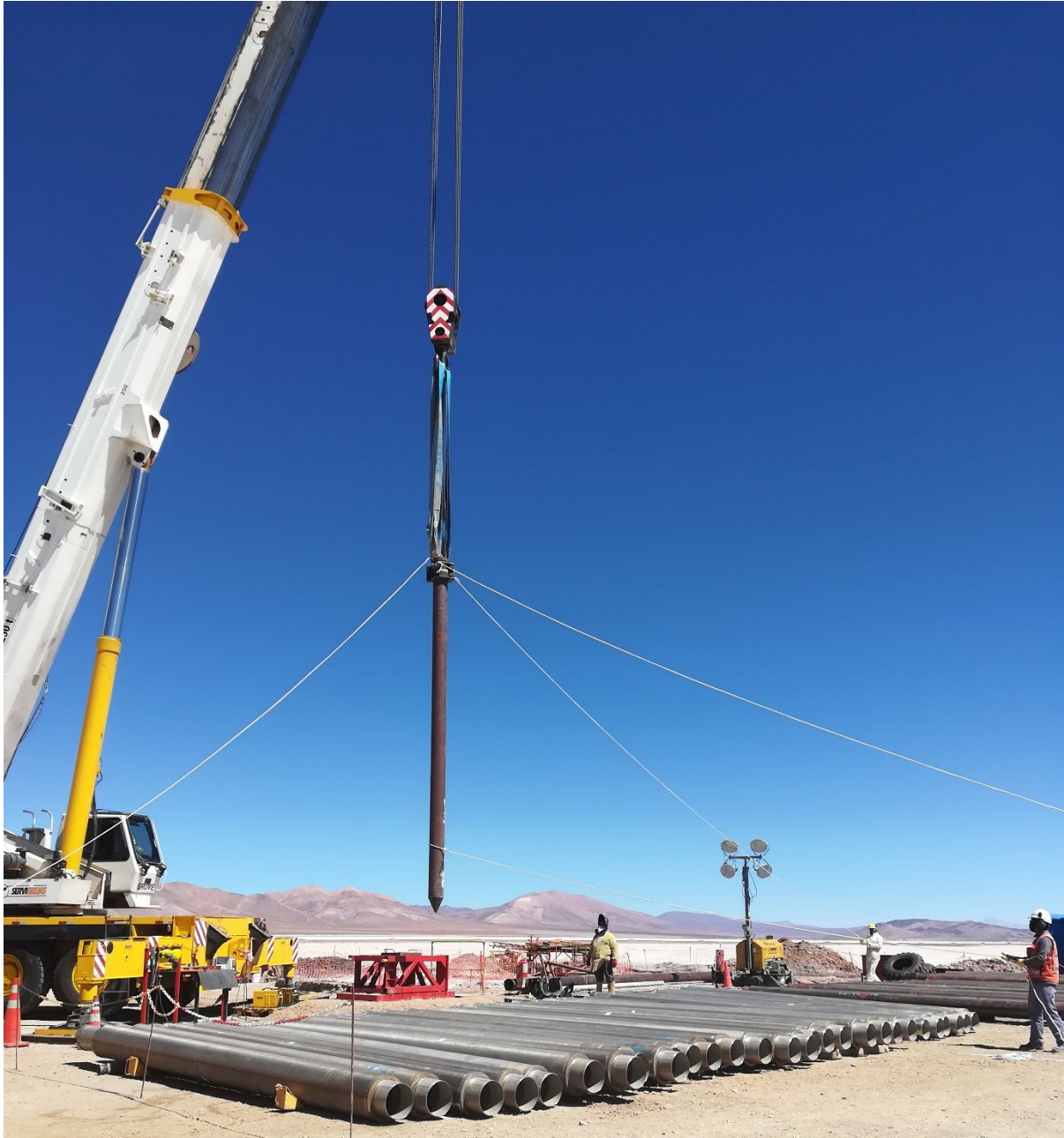
Figure 10.3: Installation of filters in a production well at the Olaroz Project
