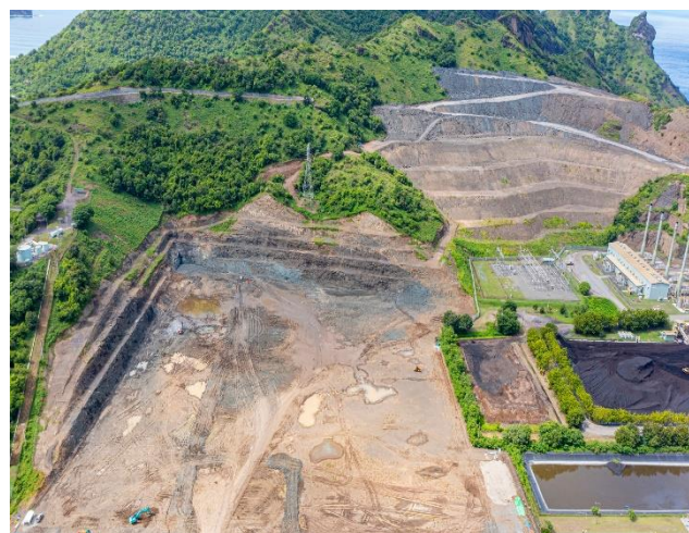
Combined cycle power plant progress
