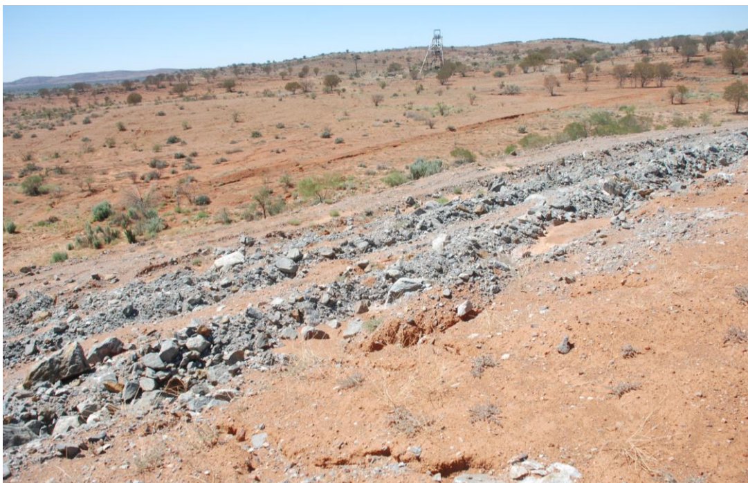
Plate 5 Contour ripping and integration of growth medium into underlying waste rock material on the eastern Potosi WRE batter
