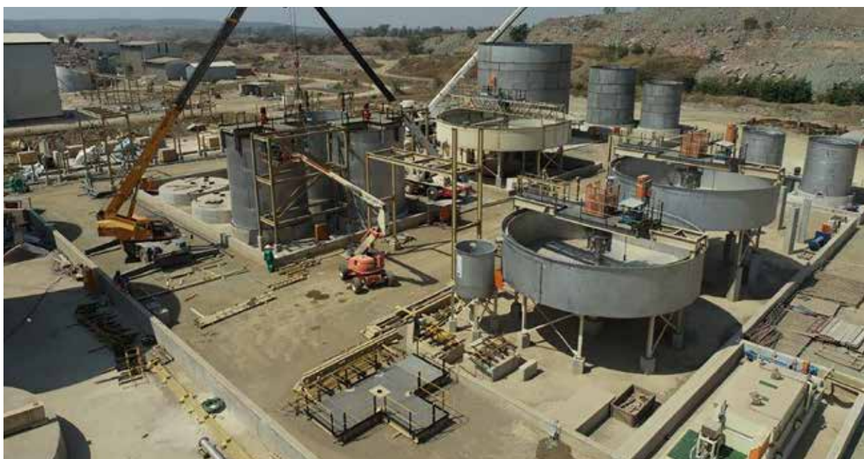
BIOX Plant under construction
