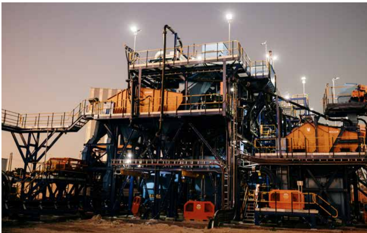
Part of the Crown Jewel plant project
