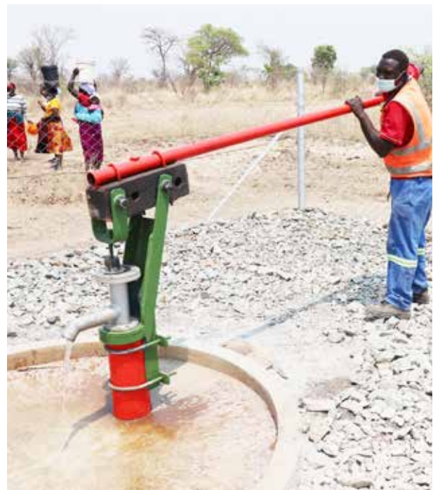
Commissioning of Community Borehole in Chakari Area
