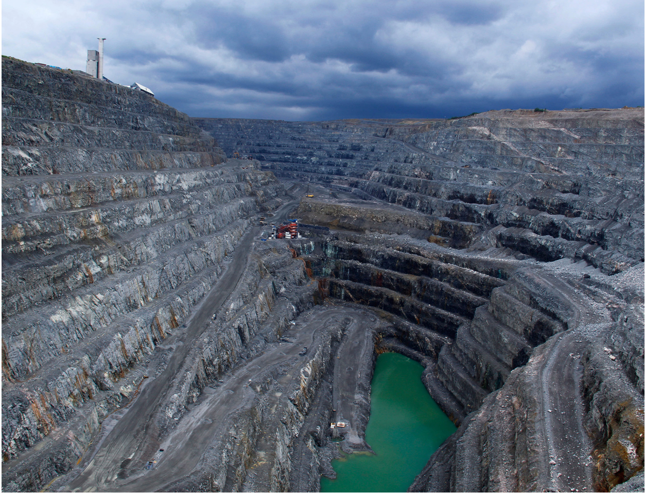
Swedish ore production has almost doubled over the past ten years. Much of the increase is attributable to the Aitik mine. Photo: Boliden
