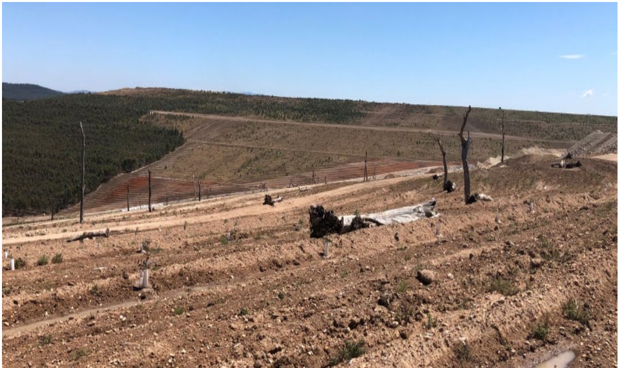
Figure 14 - Photo: Salvaged trees laid down and erected in the Northern Rehabilitation area in 2020
