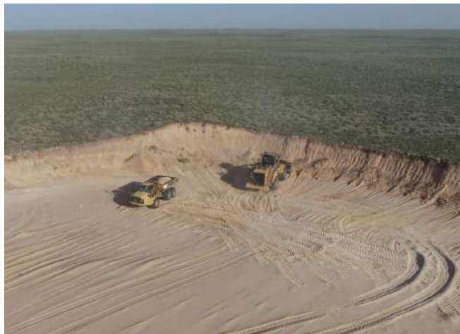
Figure 13.1: Loading Operations at the Lamesa Operation
