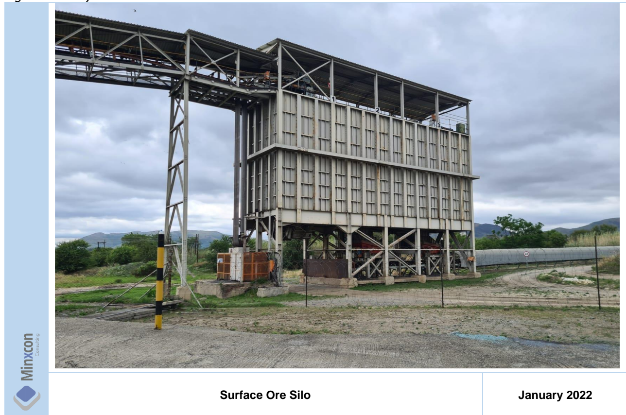
Figure 82: Surface Ore Silo
