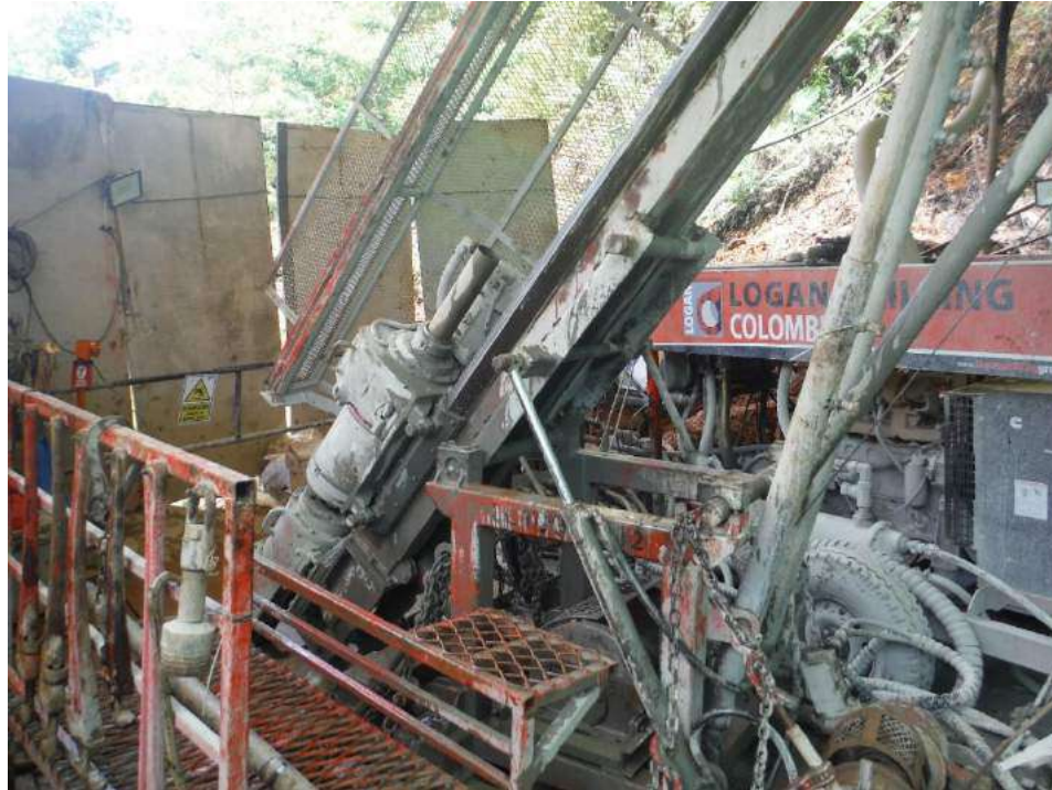
Figure 12.1 – Example of Drilling Validation
