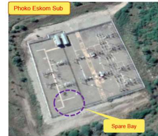
Figure 5-14: Phoko Substation and OHL
