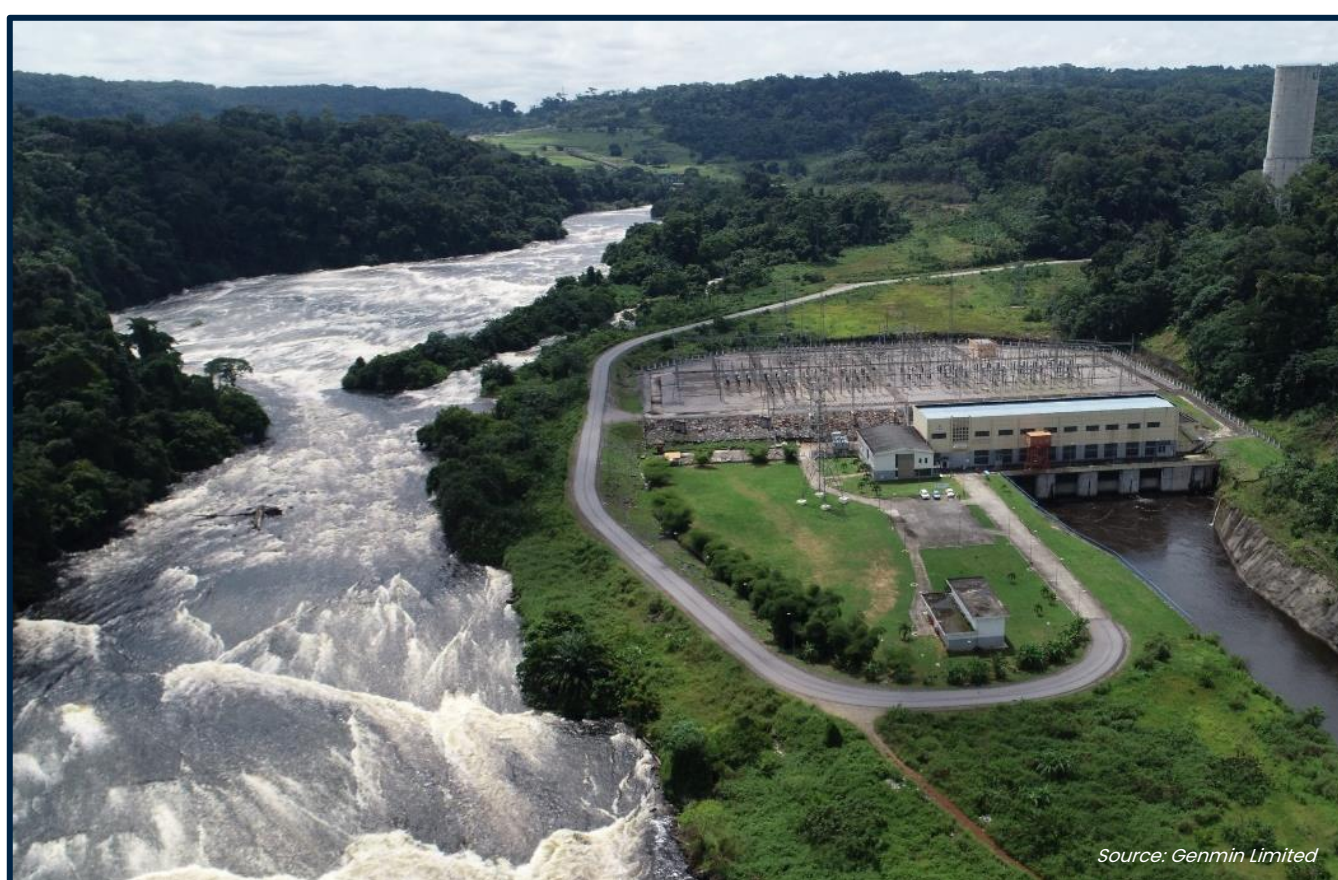
Figure 14: Aerial view of the Grand Poubara Hydroelectric Power Station
