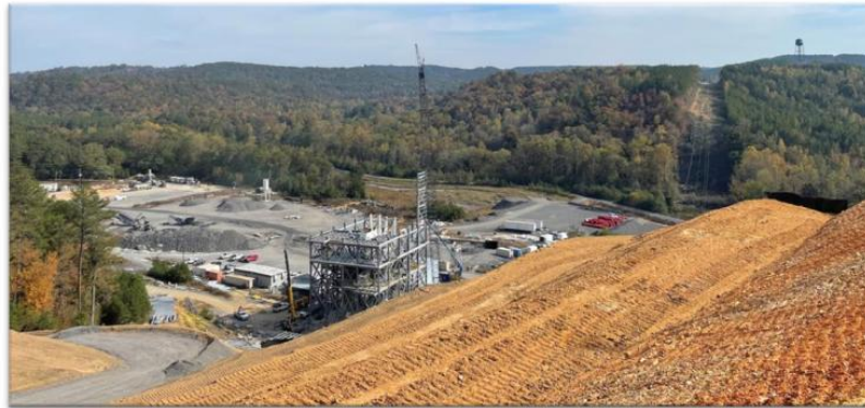
Figure 2-1: Blue Creek Mine Construction Site (October 23, 2023)
