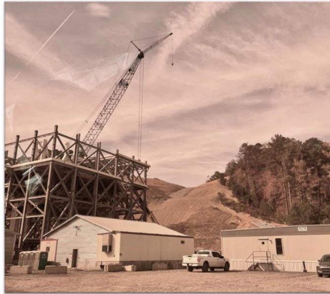
Figure 2-2: Blue Creek Mine Construction Site (October 23, 2023)
