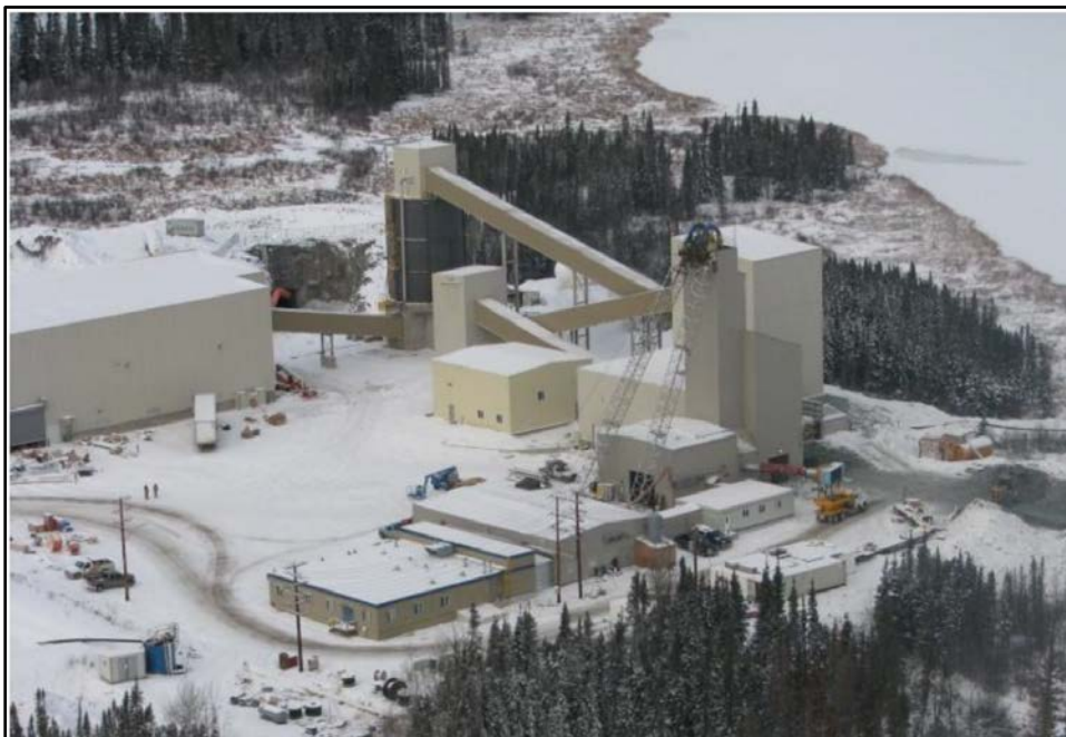
FIGURE 17.1 BUCKO PROCESS PLANT SITE, 2012
