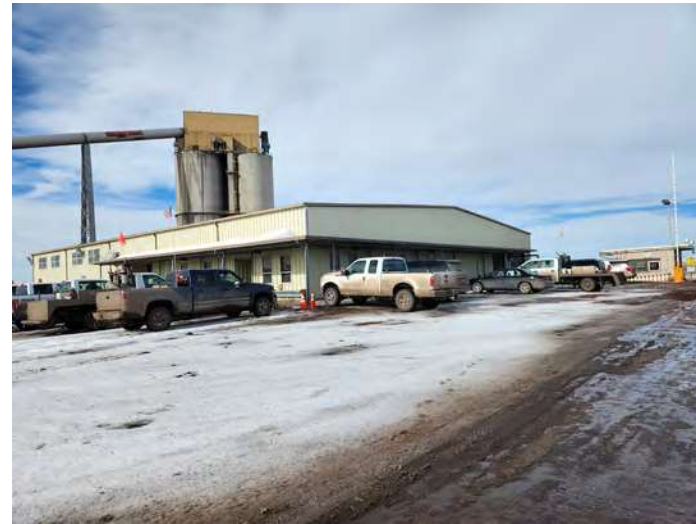
#1 GUARD SHACK & OFFICE
