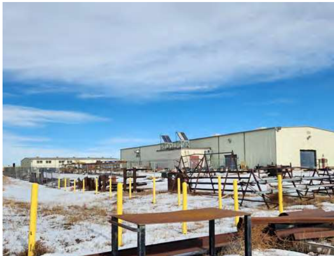
#8 WAREHOUSE & LIGHT DUTY SHOP, FENCED STORAGE
