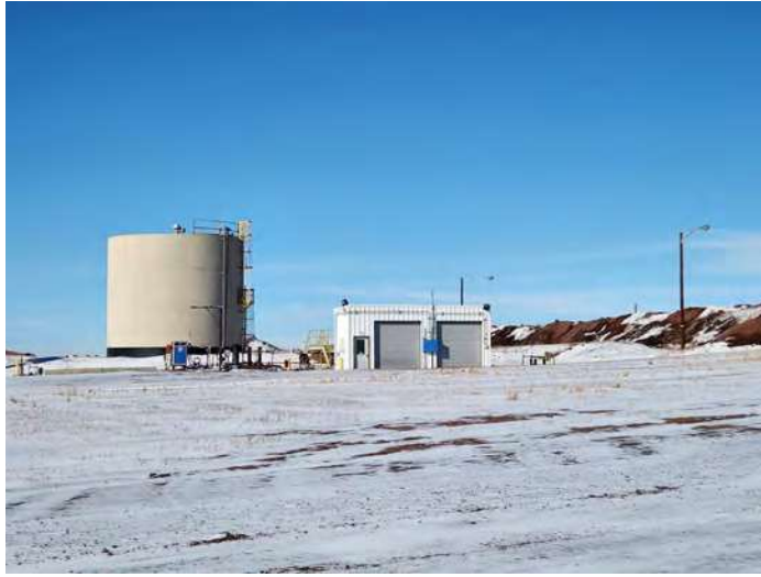
#19 BULK FUEL STORAGE & DISPENSING
