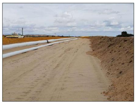
▲ Figure 11: Example of secondary containment to be constructed for all pipelines.
