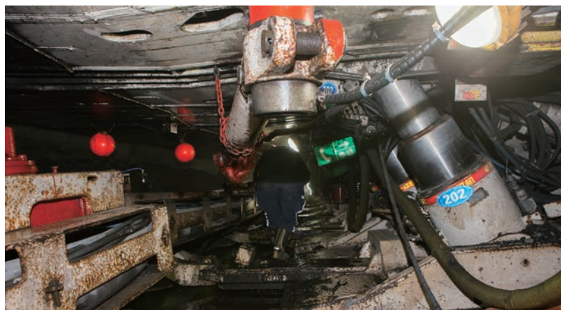
New technology of automatic coal cutting in intelligent fully mechanized face
