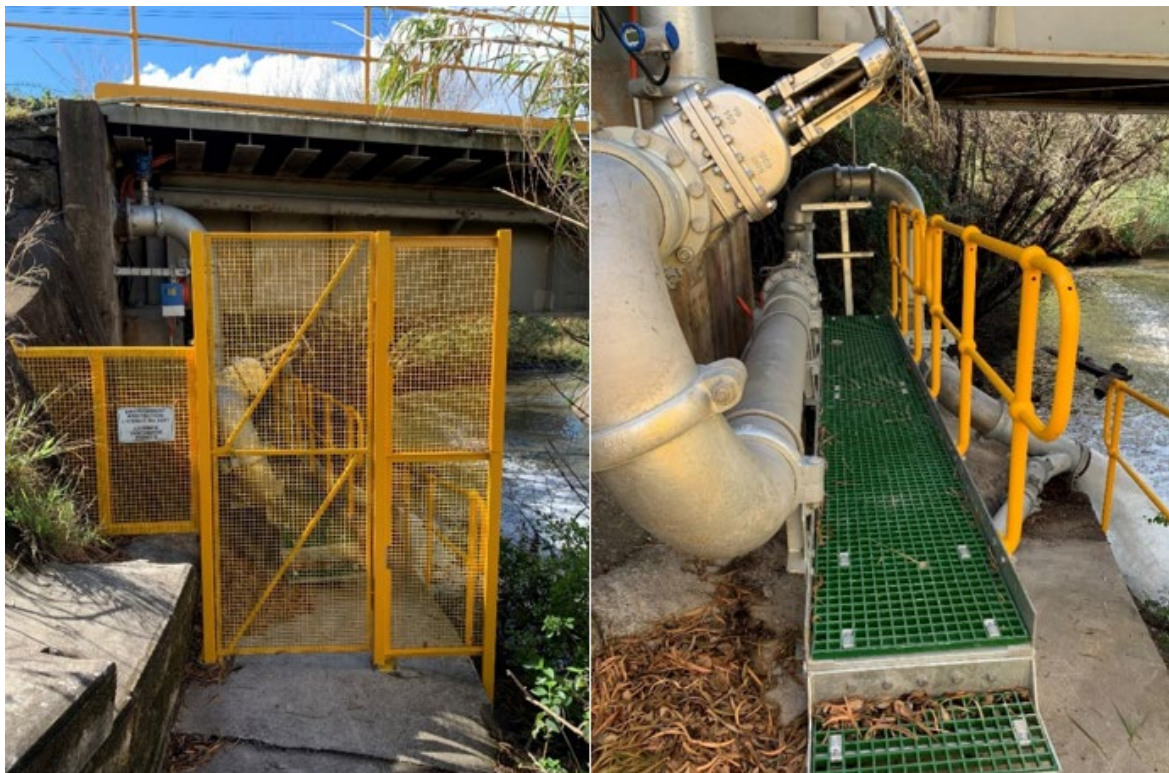
Plate 5: LDP 5 access gate (left) and walkway (right)
