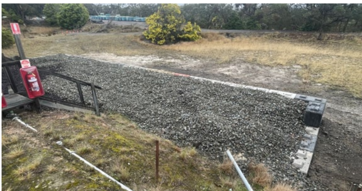
Plate 6: New retaining wall behind Primary Separation Lagoon at Cordeaux Colliery
