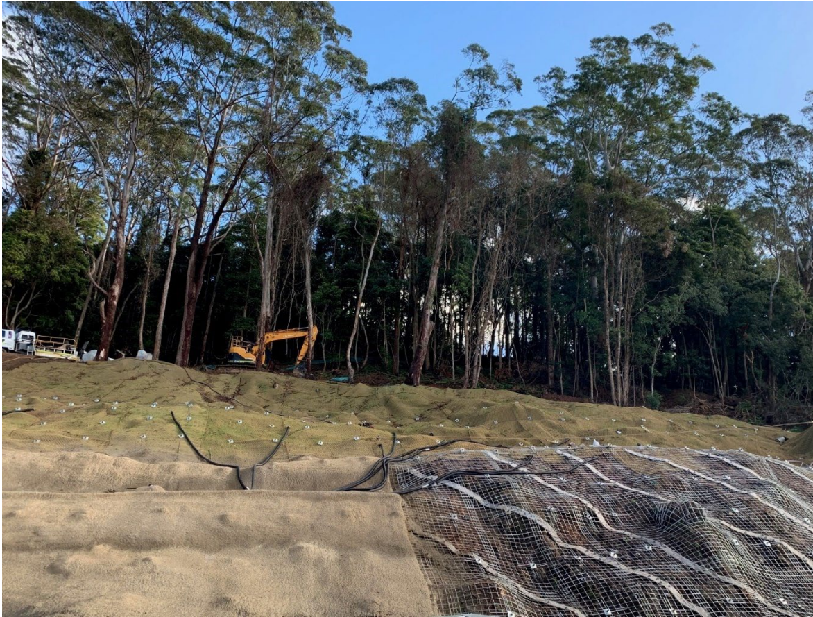
Plate 3: Slope Remediation Works - Dendrobium Pit Top
