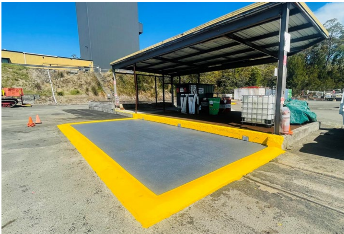
Plate 9: Newly constructed bunding of diesel filling point, Cordeaux Colliery
