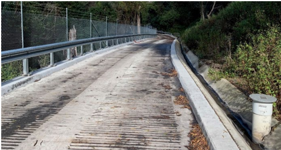
Plate 1: Lower Portal Road Upgrade
