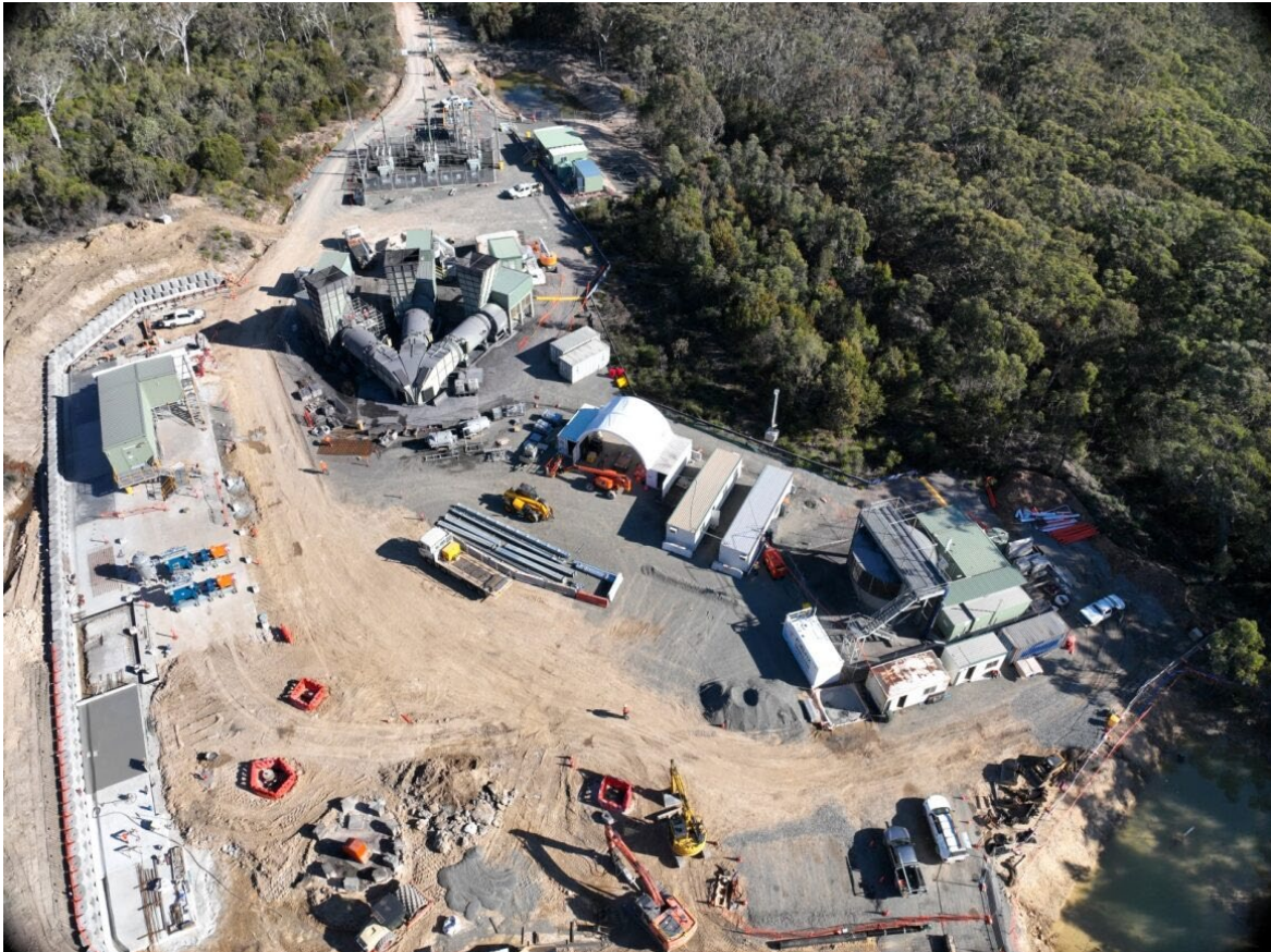
Plate 4: Gas Management Infrastructure Progress - July 2023
