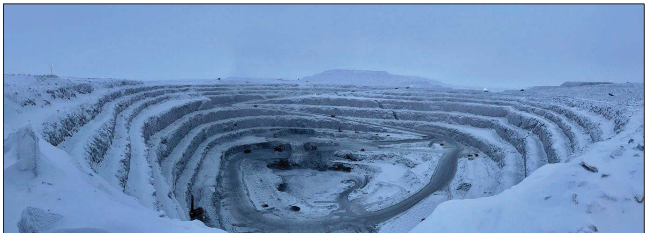
Figure 9-9: Aerial view of Sable pit, 2022
