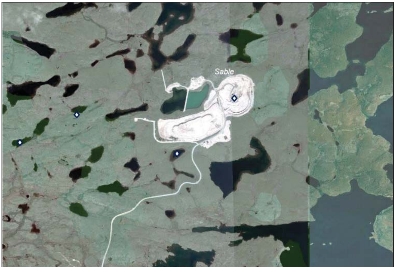
Figure 9-4: Overview of the Sable open pit area
