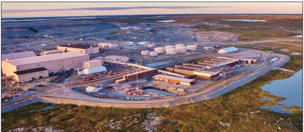
Figure 3-3: Ekati Diamond Mine infrastructure
