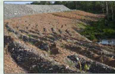
Figure 34 | Rehabilitated batter on waste dump
