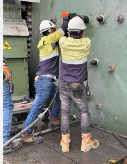
Figure 3 | Okvau Maintenance Personnel
