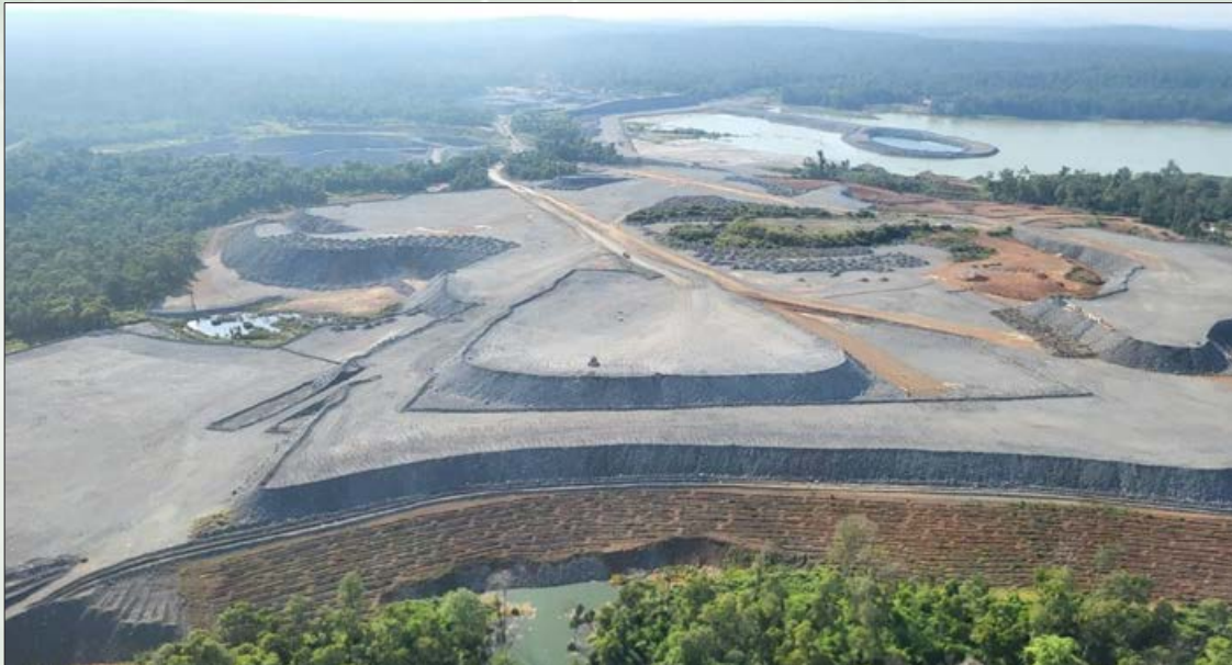
Figure 28 | Okvau’s tailings dam and waste dumps
