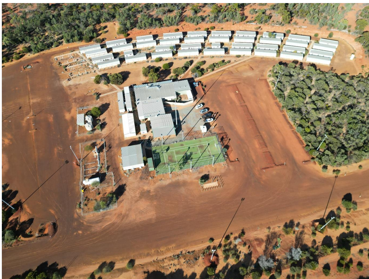
Image 9: Extension Hill Camp Infrastructure
