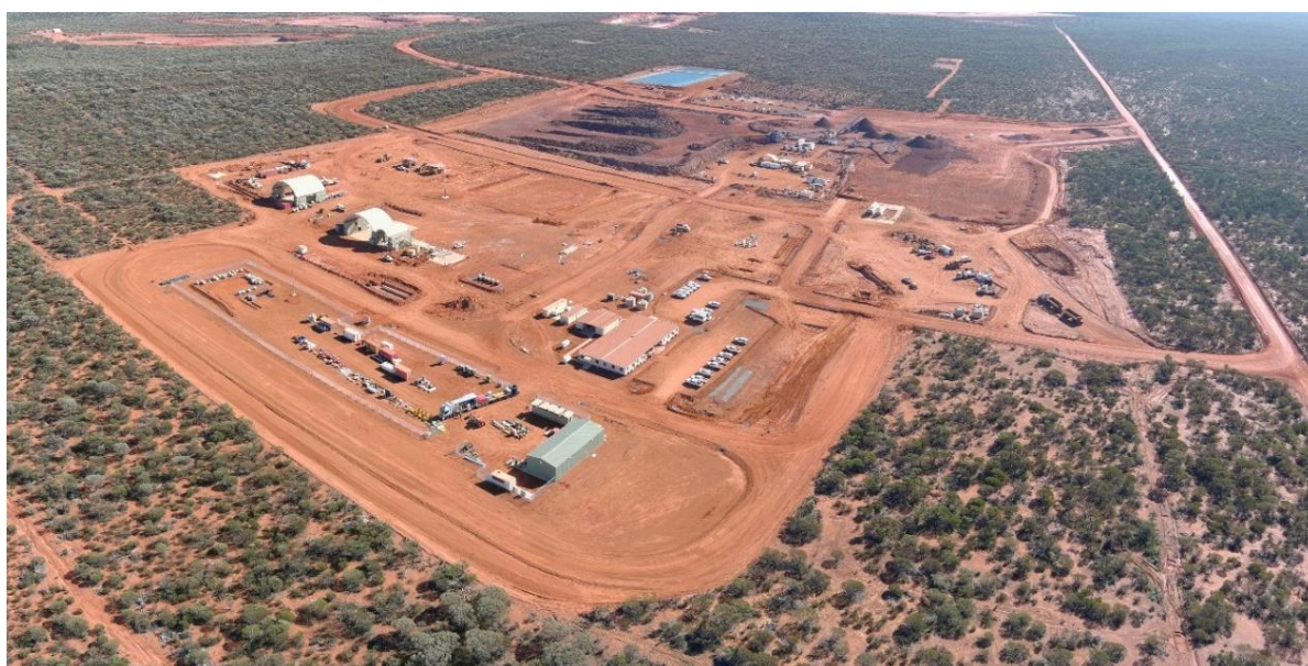
Image 2: The Shine Iron Ore Mine – Infrastructure and Crushing Area July 2021
