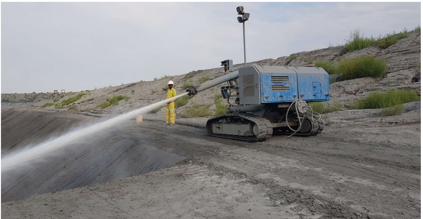
Figure 18: Semi-automated, track mounted, top-down hydro-mining in operation (Source: Paragon)
