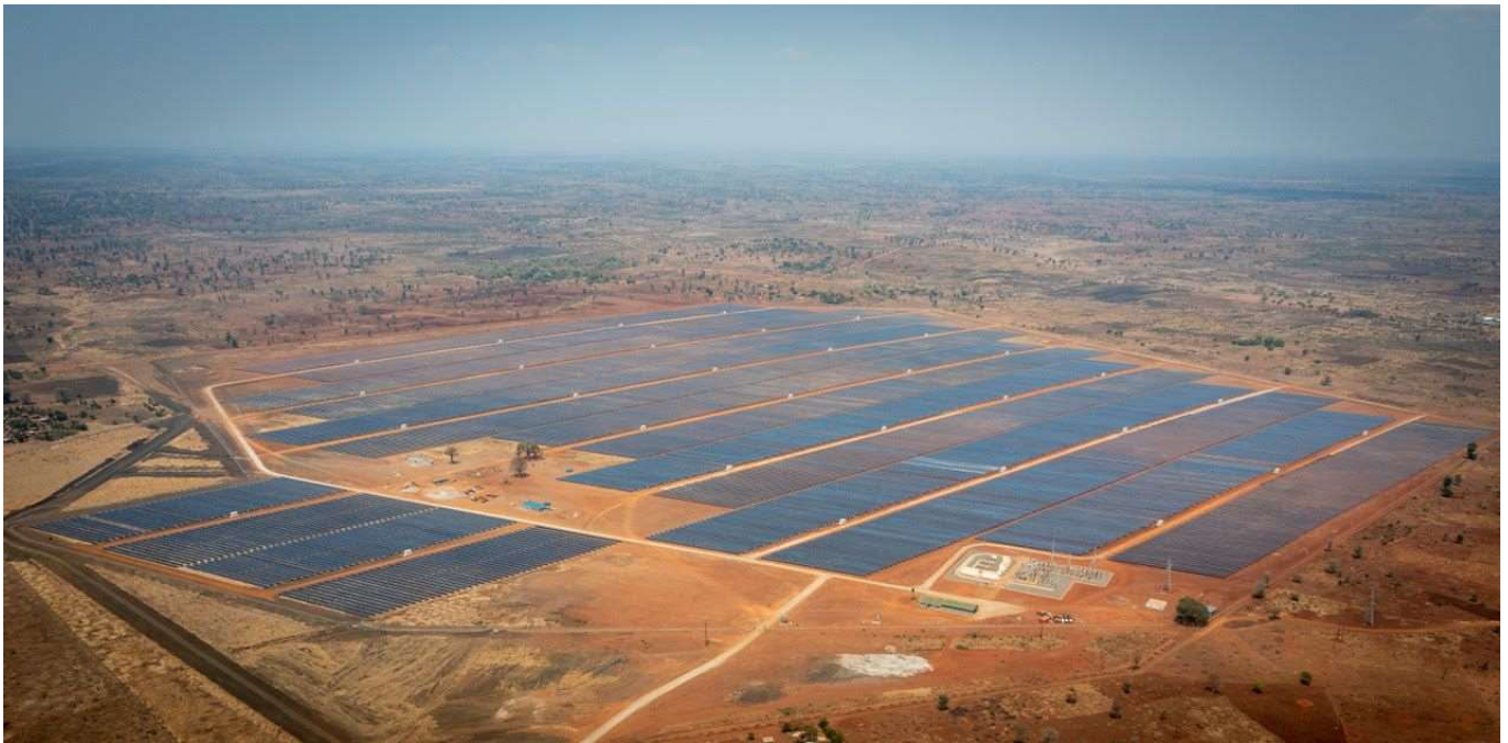
Figure 31: 60MW Salima Solar Power Plant in Malawi recently constructed and commissioned by JCM (source: JCM)
