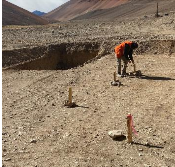
Figure 12.2: Drill Pad Preparation
