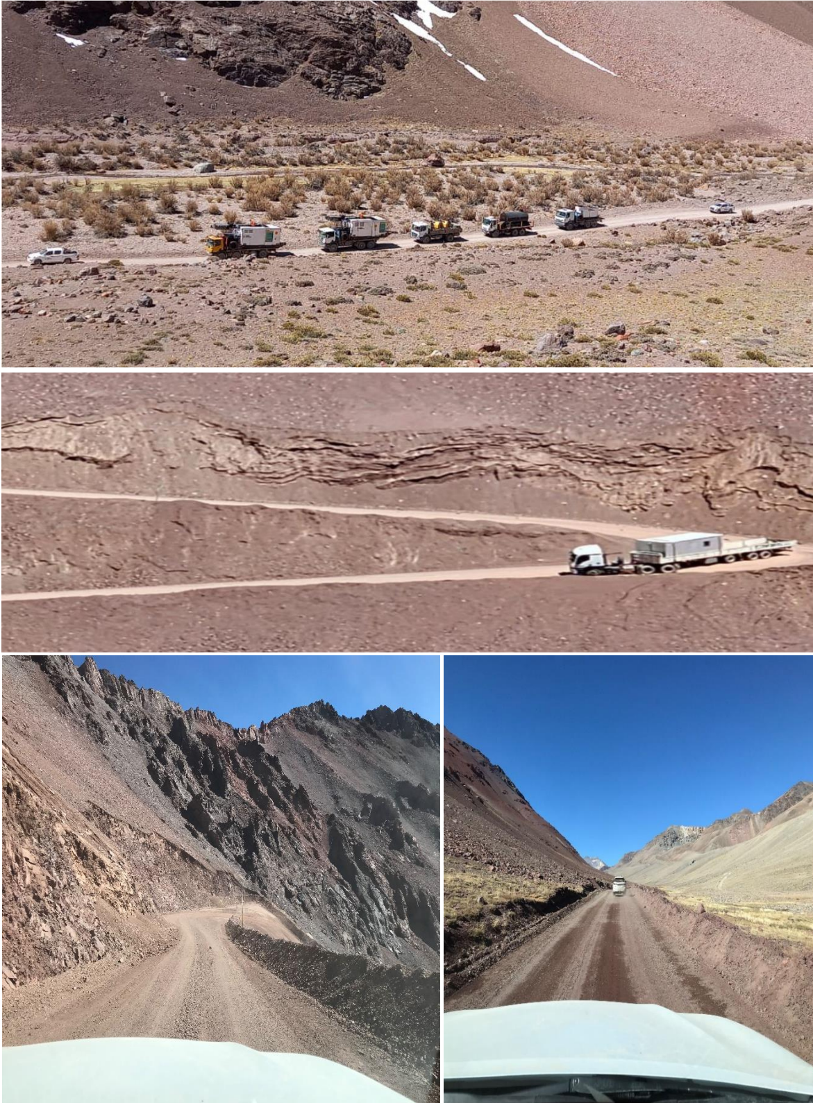
Figure 18.3: Access Roads Photos (McEwen, 2023)
