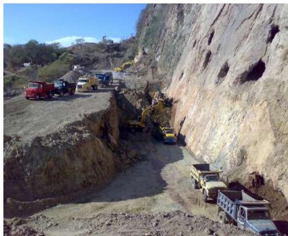
A.) LOOKING NORTHWEST ALONG EL ABRA WORKINGS
