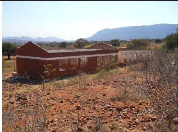
Fig 74. Abandoned school ruin near sites 1 – 3.
