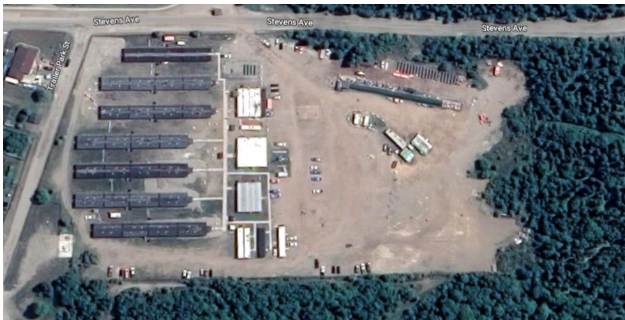
Figure 18.27: Marathon Construction Camp
