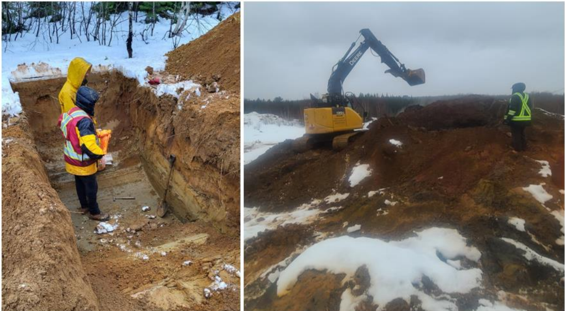
Figure 9.3: Typical test pit excavations
